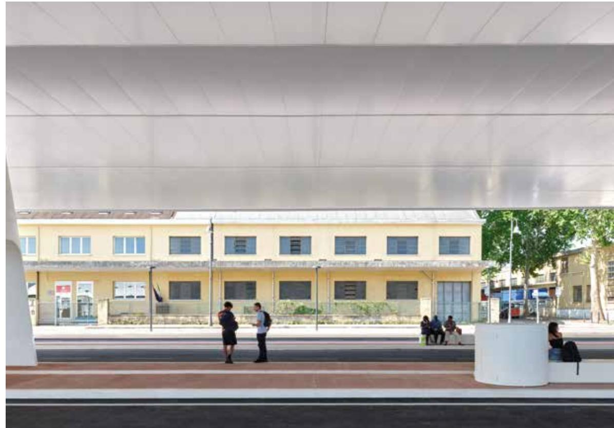
Constructed in steel and aluminum, the canopy of the new Bus Terminal in Cesena is supported by four inclined conical steel pillars, each weighing 30 tons, which enhance the sense of dynamic tension and controlled instability, while ensuring structural efficiency. Combining functional efficiency with formal ambition, the project transforms a space of transit into a powerful architectural statement. The precise, linear geometry of the structure resonates with
